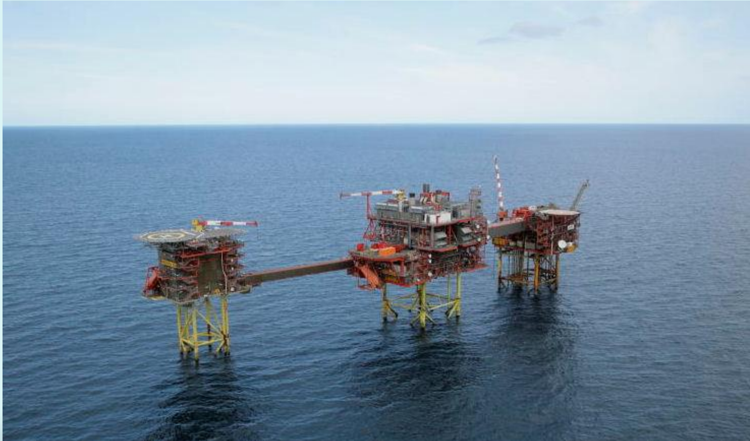
ConocoPhillips Murdoch platform complex in 37m water depth
