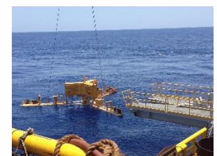
Photos courtesy of FMC Technologies
